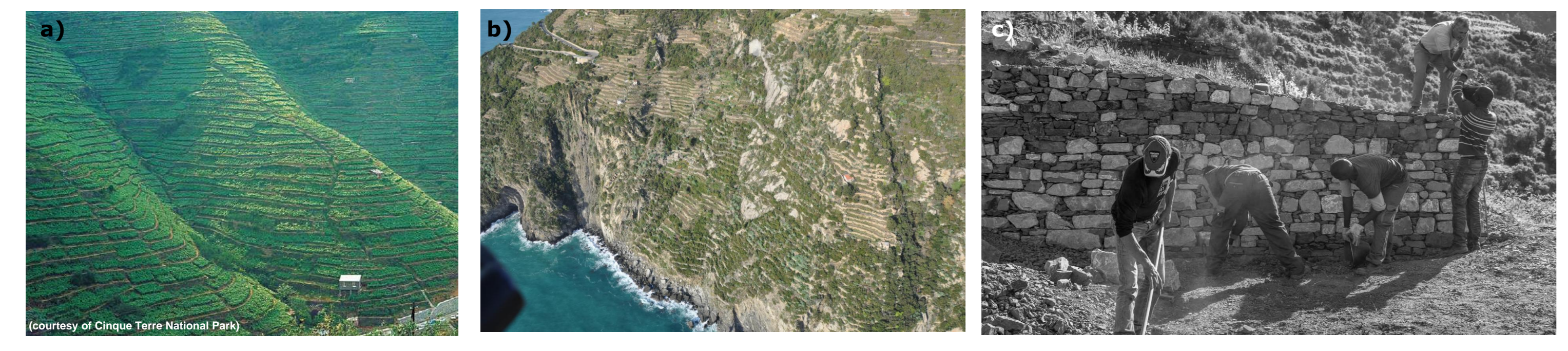
Fig. 1 (a-b) Terraced slopes along the coast of Cinque Terre (Italy); (c) dry-stone walls construction activities.
