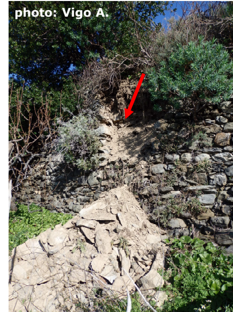
Dry-stone walls deformations & collapses
