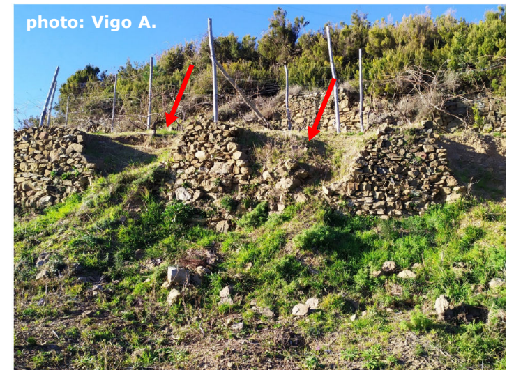
Dry-stone walls deformations & collapses
