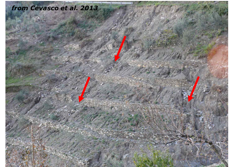
Terraced slope affected by rill erosion
