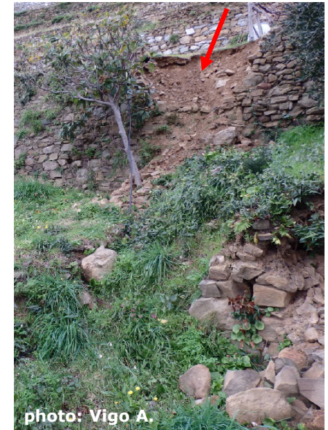
Dry-stone walls deformations & collapses
