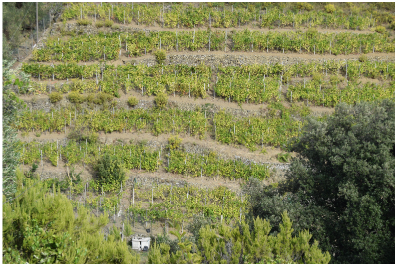
Terraced slopes with terraces sustained by dry-stone walls in Cinque Terre (Italy)
