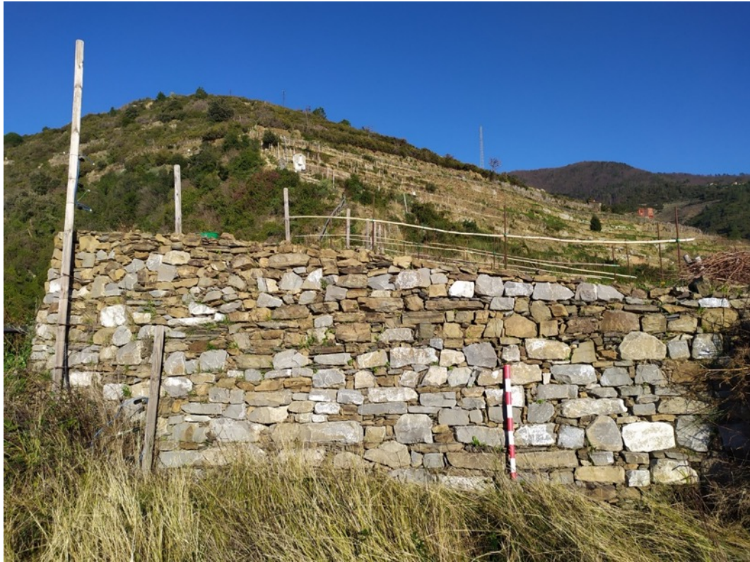
Figure 18 Dry-stone wall reconstructed with autochthonous and allochthonous materials.
