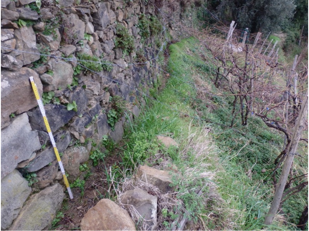
Figure 14 A maintained drain channel
